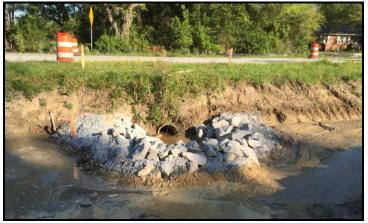
Sediment Dam for Pipe Inlet
