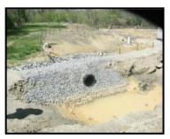
Pipe Slope Drain Inlet with Berm
