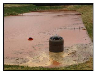
Temporary Surface Outlet and Baffle Sediment Basin
