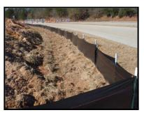
Silt Fence with Steel Post
