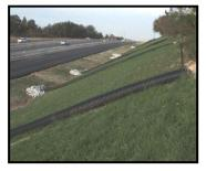
**Pipe Slope Drains**
