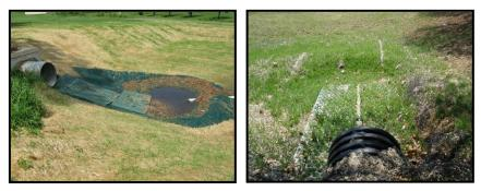
Level Spreader for Outlet Protection
