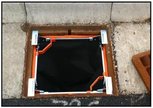
Type G Suspended Internal Inlet Filter
