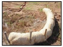
Sediment Tube for Ditch Check
