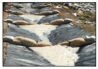
Passive Flocculant Treatment System with Sediment Tubes (Photo Courtesy of Clemson University)
